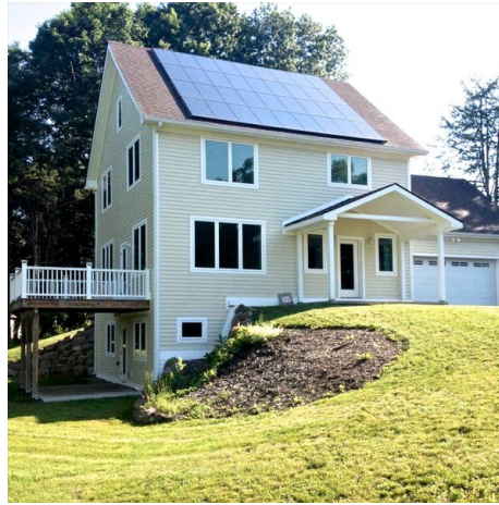
A "net-zero" house in New York. Between the solar panels and geothermal pumps, the house essentially produces as much energy as it consumes. The proliferation of distributed technologies is impacting the way New York will plan and design its bulk power system. Source: Greenhill Contracting
